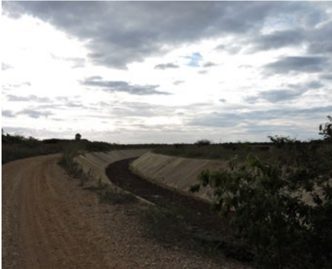
Construction for the São Francisco River diversion. (Credit: Luiz Felipe Lacerda.)
